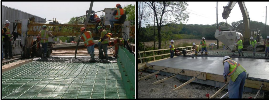
Figure 2-9: Left - Internally cured concrete being cast at Bartell Road in New York (Wolfe, 2010), and Right - Internally cured concrete bridge deck being cast near Bloomington, IN (Di Bella, Schlitter, & Weiss, 2010).
